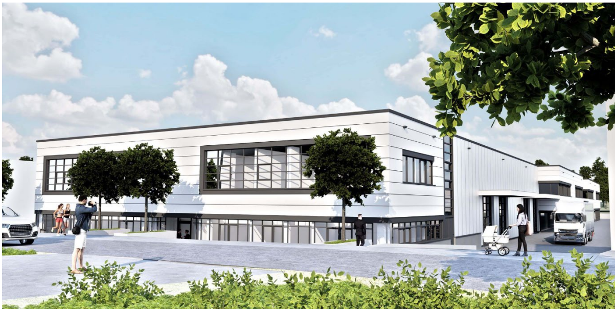
Picture 2: Construction plan for the new Pulsar headquarters: the new building complex is scheduled for completion at the end of 2024 and will offer all the prerequisites for a sustainable and attractive workplace.
